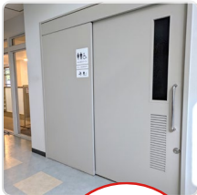
▼ Universal Toilet 2F in front of the entrance
